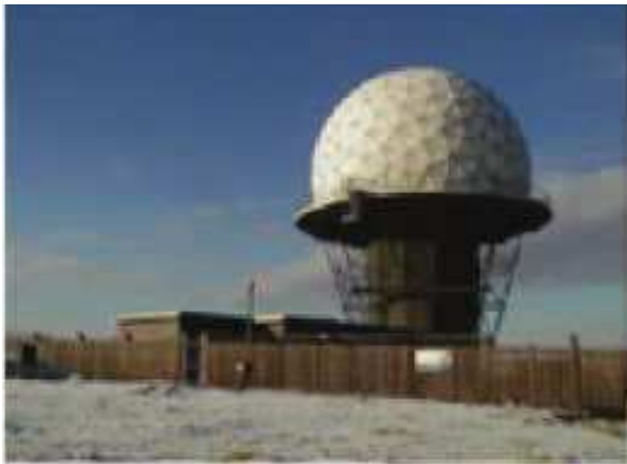
Figure 17.1 ATC radar head at Cleve Hill, Shropshire
