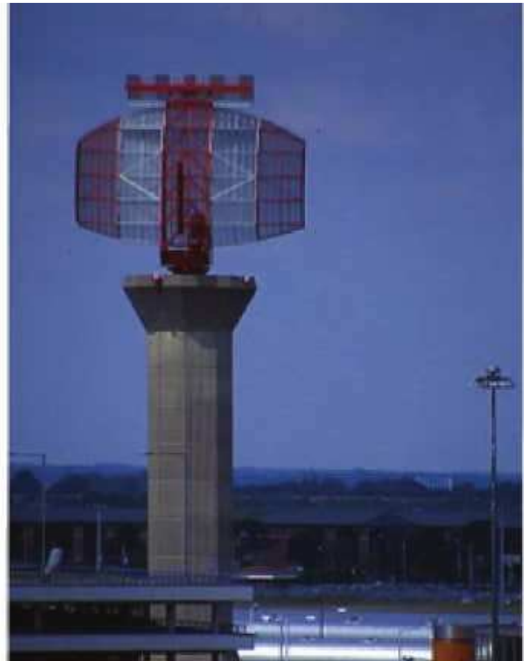
Figure 17.2 ATC radar head at London Heathrow
